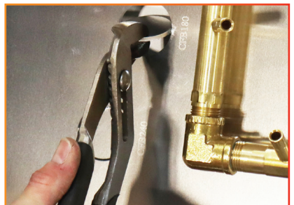
Photo 2: Breaking the Knockouts
