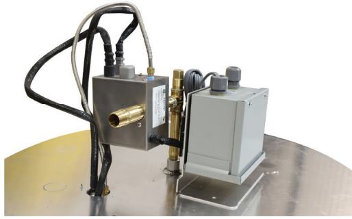
Photo 25: Connecting the 3/4" x 3" nipple to the Platinum Valve
