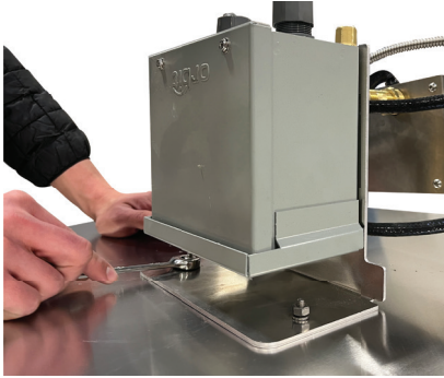
Photo 13: Mounting the Transformer to the Plate
