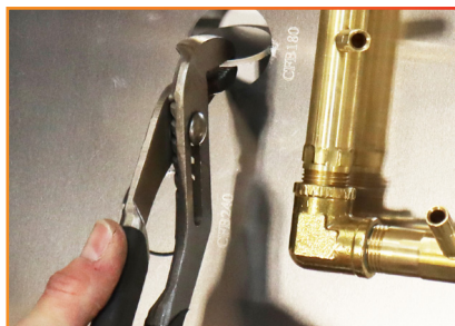
Photo 2: Breaking the Knockouts
