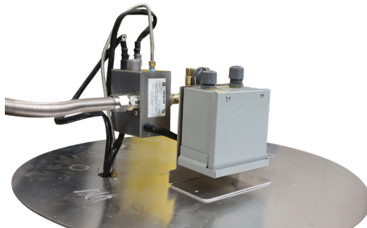
Photo 21: Attaching the Flex Line
