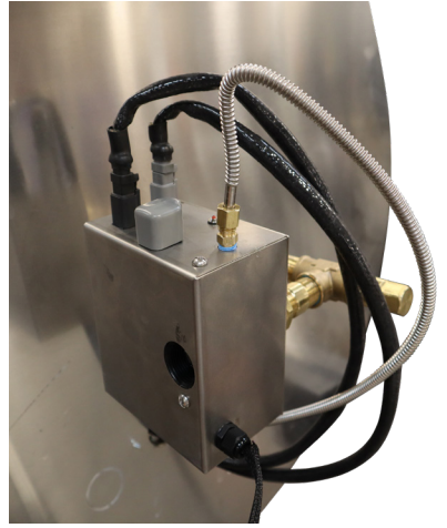
Photo 12: Connecting the Gas Line From the Pilot to the Valve
