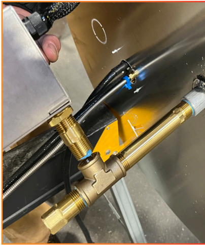
Photo 9: Attaching the Valve Box to the Drip Leg
