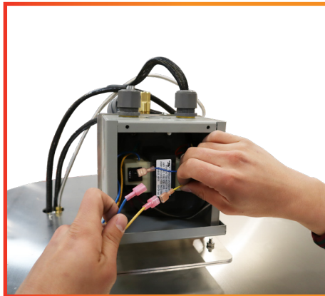
Figure 17: Connecting the Valve to the Transformer
