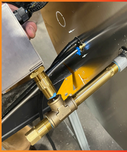
Figure 9: Attaching the Valve Box to the Drip Leg
