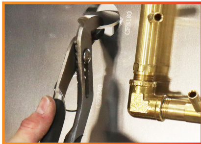
Figure 2: Breaking the Knockouts
