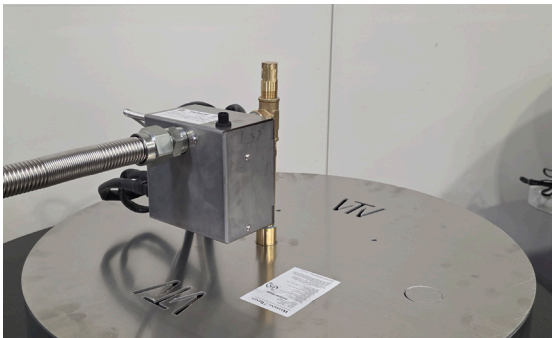
Photo 21: Attaching the Flex Line
