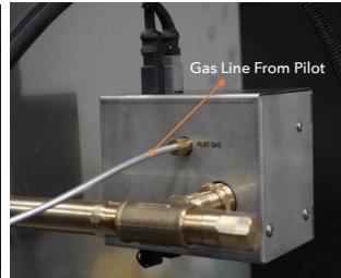
Photo 11: Connecting the Gas Line From the Pilot to the Valve
