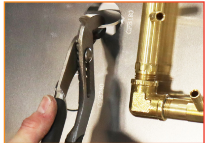
Photo 2: Breaking the Knockouts
