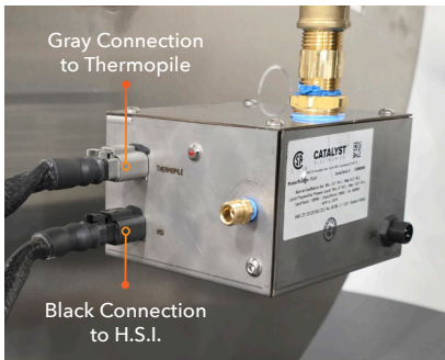
Photo 10: Electronic Connections from the Pilot to Valve
