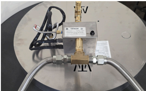
Photo 27: Connecting the Flex Lines to the Flared Fittings
