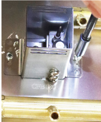
Photo 5: Securing the Pilot to the Plate/Pan
