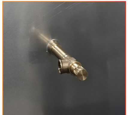
Photo 7b: Installing the Drip Leg
