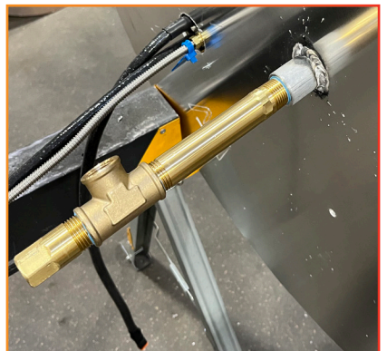
Photo 7b: Installing the Drip Leg
